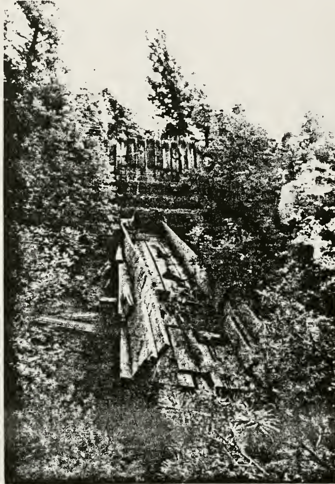
Figure 251. Feature #142, ore bins and gravity ore chute, east view.
